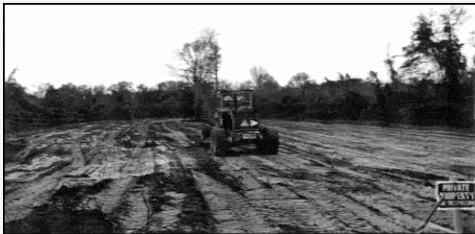
Mechanical stripping at James City Site
